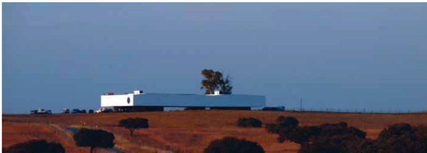
Garducho Biological Station - Mourão, PORTUGAL (Systems ETICS and FacadeS with cork at sight)
