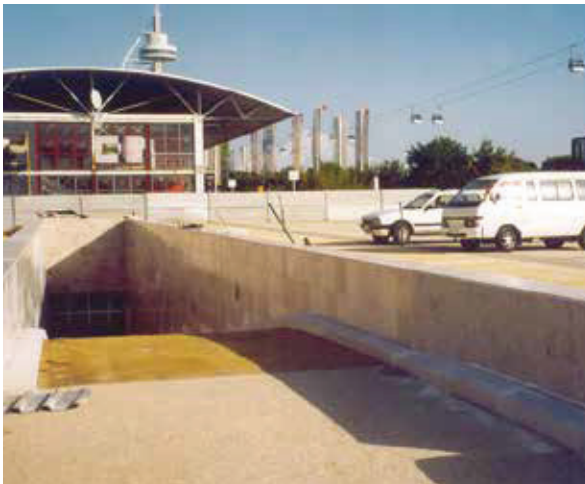
Tágides Car Park - Lisbon, PORTUGAL (Light weight concrete)
