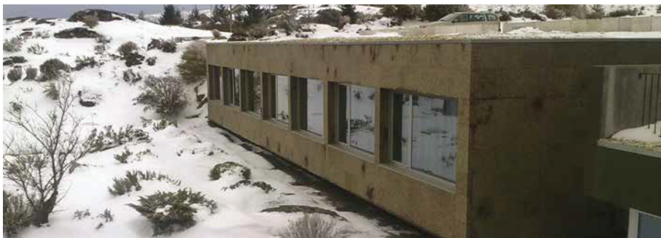
Hotel Penhas Douradas - Serra da Estrela, PORTUGAL (System ETICS with cork at sight)
