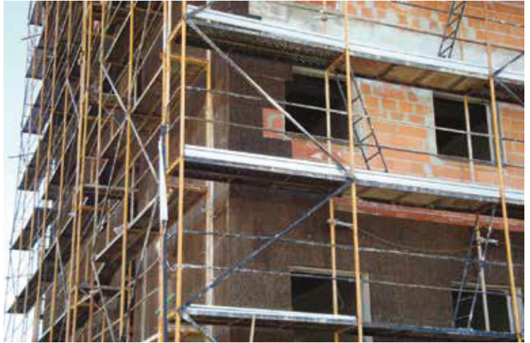
Residential Building - Santarém, PORTUGAL (System FACADES)
