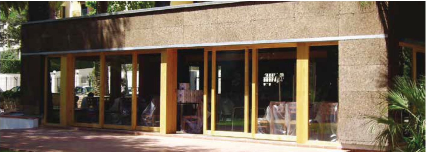
Bar - Estoril, PORTUGAL (System ETICS with cork at sight)
