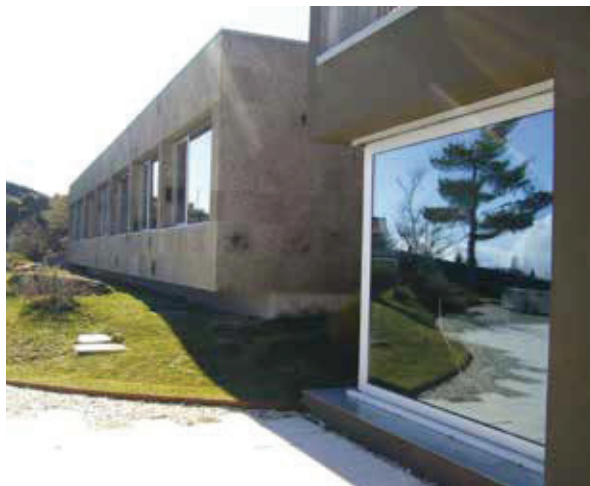
Hotel Penhas Douradas - Serra da Estrela, PORTUGAL (System ETICS with cork at sight)
