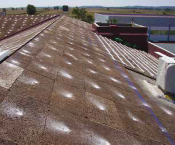
Golegã Sports' Training Centre - Golegã, PORTUGAL (Sloping roof insulation)
